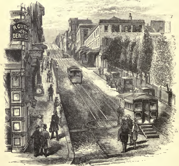
VIEW IN CLAY-STREET, Showing the dummy cable car.
